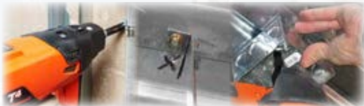
Clip Assembly to Concrete or CMU Block
